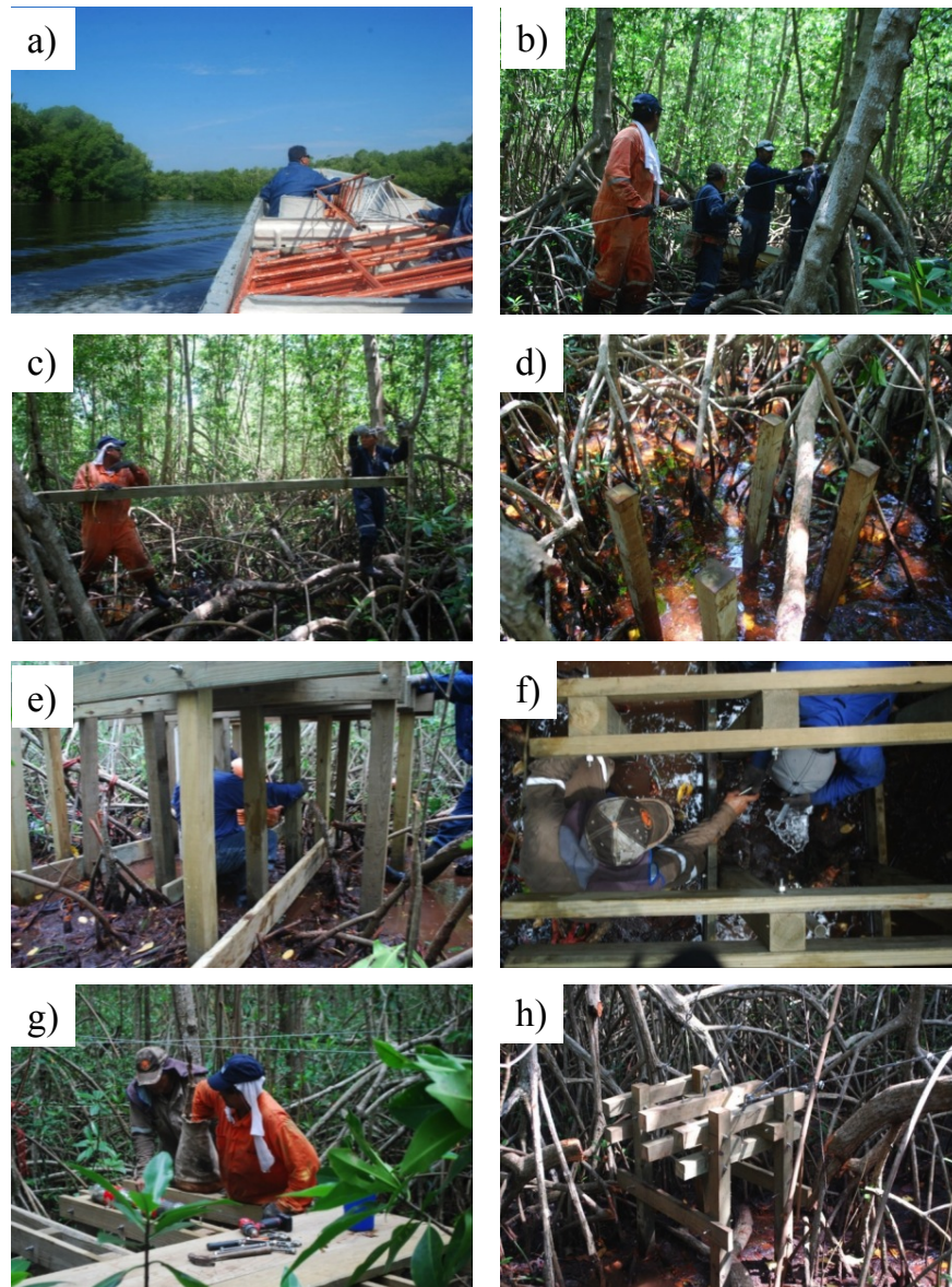
Figure 11. Main steps for installation of the tower; a) boat transport; b, c) transportation of materials; d-h) construction of the base to install the radio-tower.
